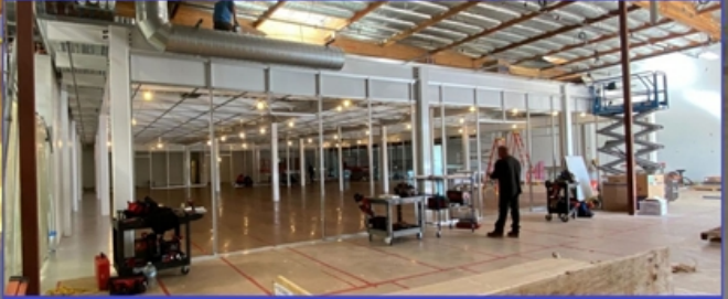
Expansion in progress
